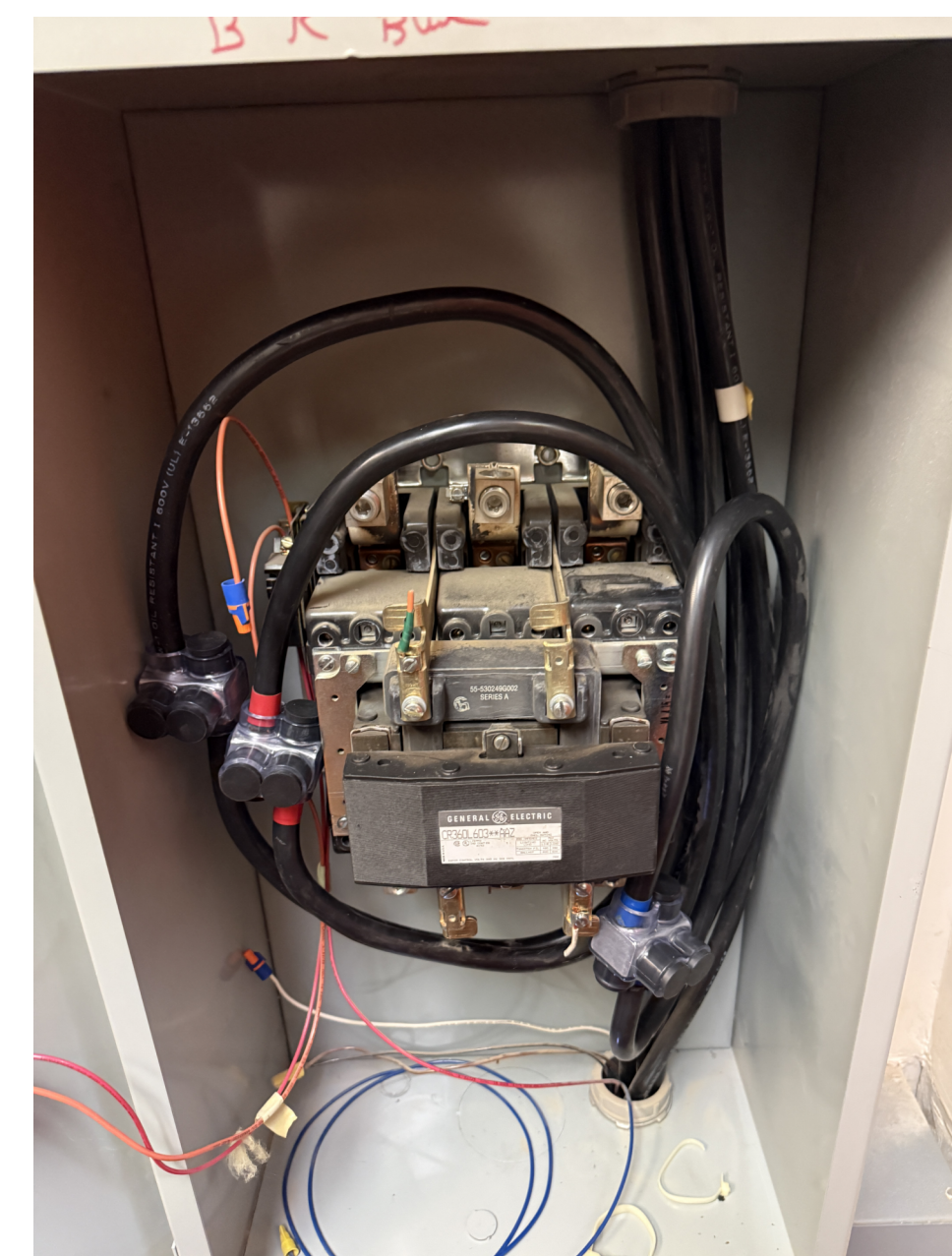
2 DETAIL IMAGE - CONTACTOR N.T.S.
